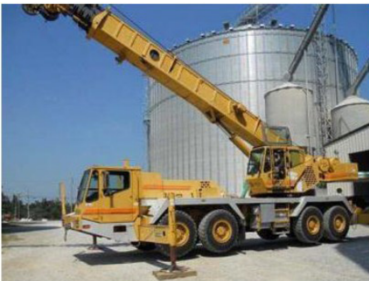
Figure 3. All-terrain, mobile, 50 ton crane.
